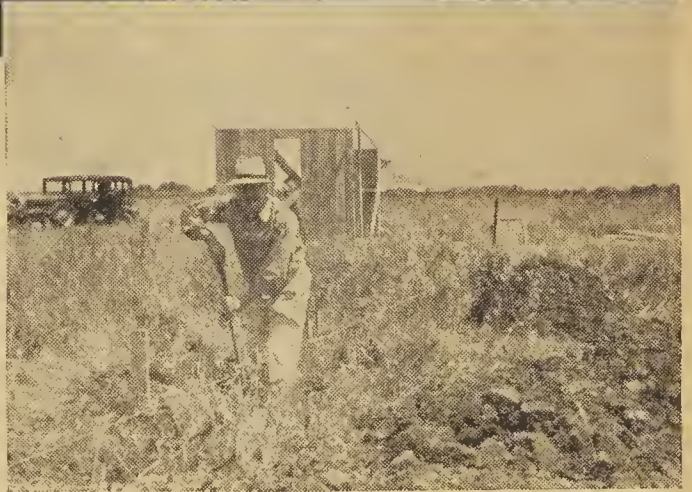
This is the beginning. I felt safer on the ground digging than I would on the tower.
